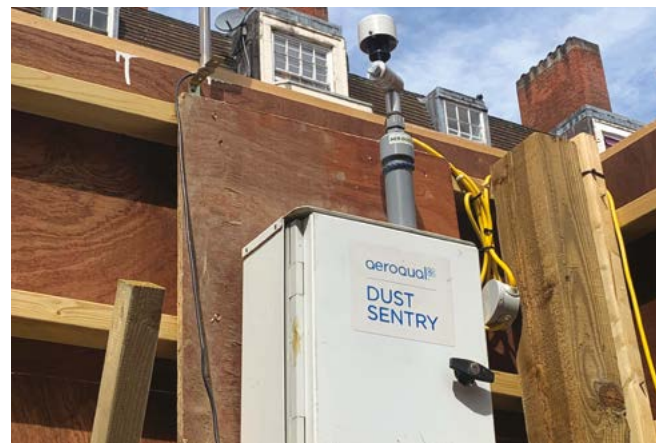
Some of our monitoring equipment
