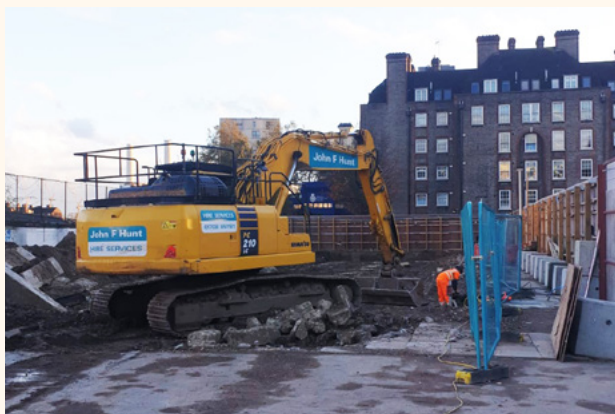
Construction work progresses at Ebury
