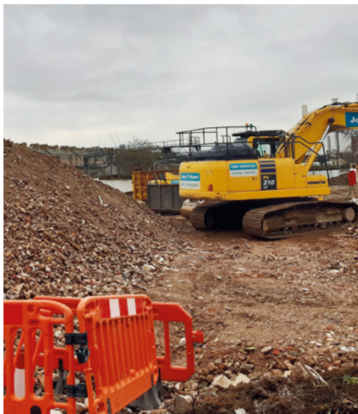
Work progresses at Ebury
