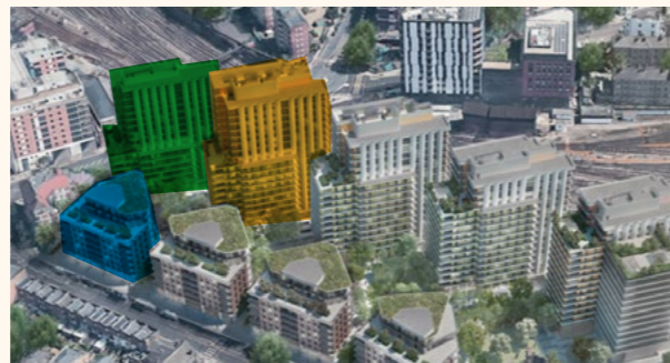
Phase 2A building area and public consultation in December 2021
