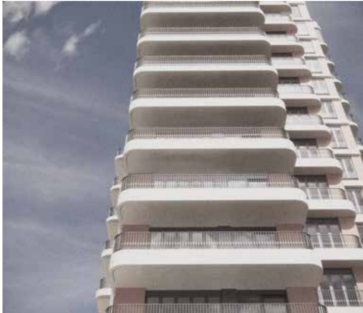
External view - Facade Zone 3 facing the railway
