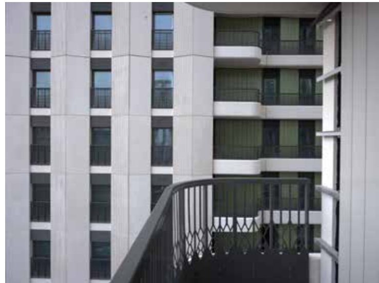
View from private balcony, looking towards adjacent building. This is a photo from the construction of Phase 1; this same detailing will apply to phase 2 Buildings 5 & 6
