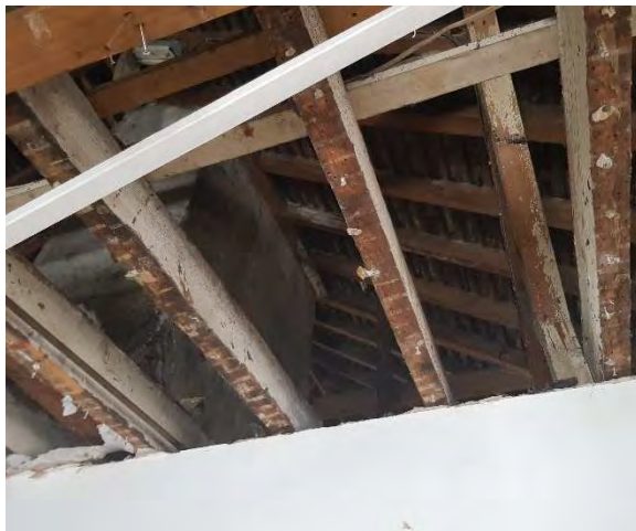
Photograph 8: Dalton House roof void. Boarding at the base on the northern side of the roof. A concrete chimney stack to the right of the picture couldn't be inspected where it meets the roof.
