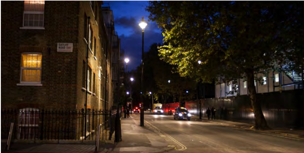
Figure 3 - Ebury Bridge and Ebury Bridge Road – 8m columns, 2800K warm white light.
