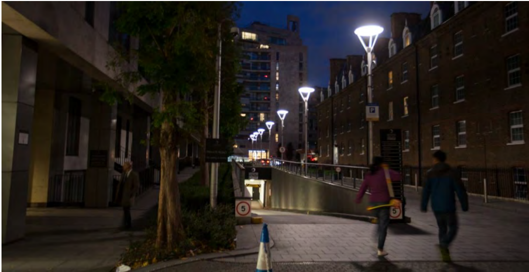
Figure 1 - Grosvenor Waterside – ca. 6m columns, indirect light, 4000K neutral white light.
